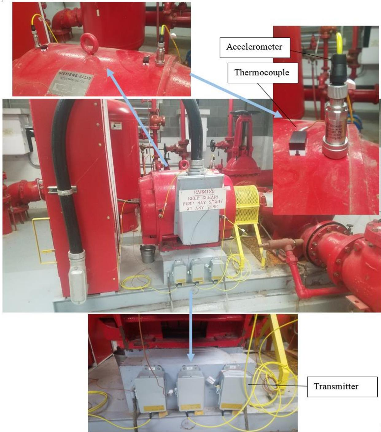
Figure 12. Vibration and temperature sensors and MSMU installation on the fire protection pump.
