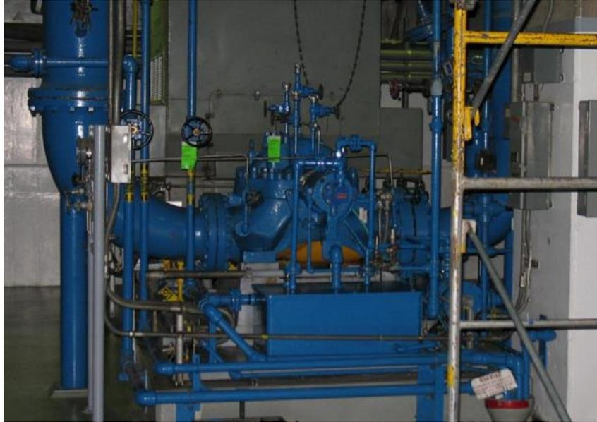
Figure 17. Condensate booster pump at Cooper Nuclear Station.
