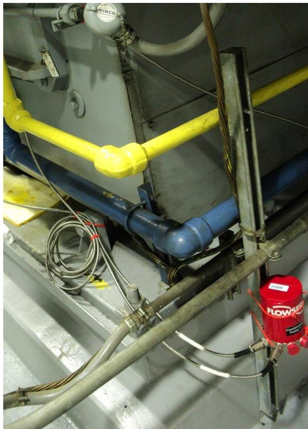
Figure 21. Installation of continuous-monitoring transmitter on condensate booster pumps.
