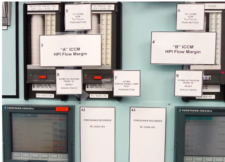
Figure 5. Photograph of paper representations of proposed display locations pasted on training simulator
