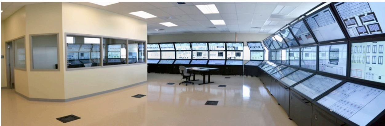
Figure 6. Photograph of glass-top simulator located in the HSSL at INL
