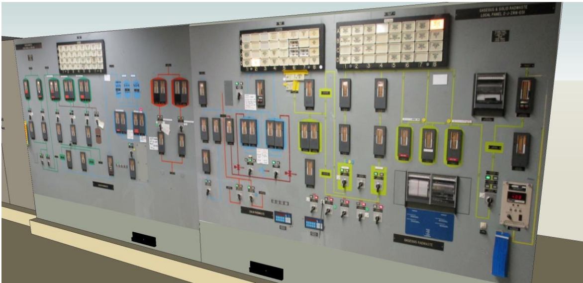
Figure 15. 3-D model of the LRS panel and gaseous and solid radiological waste panel in existing radiological waste control room.
