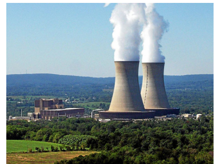
Limerick Generating Station
