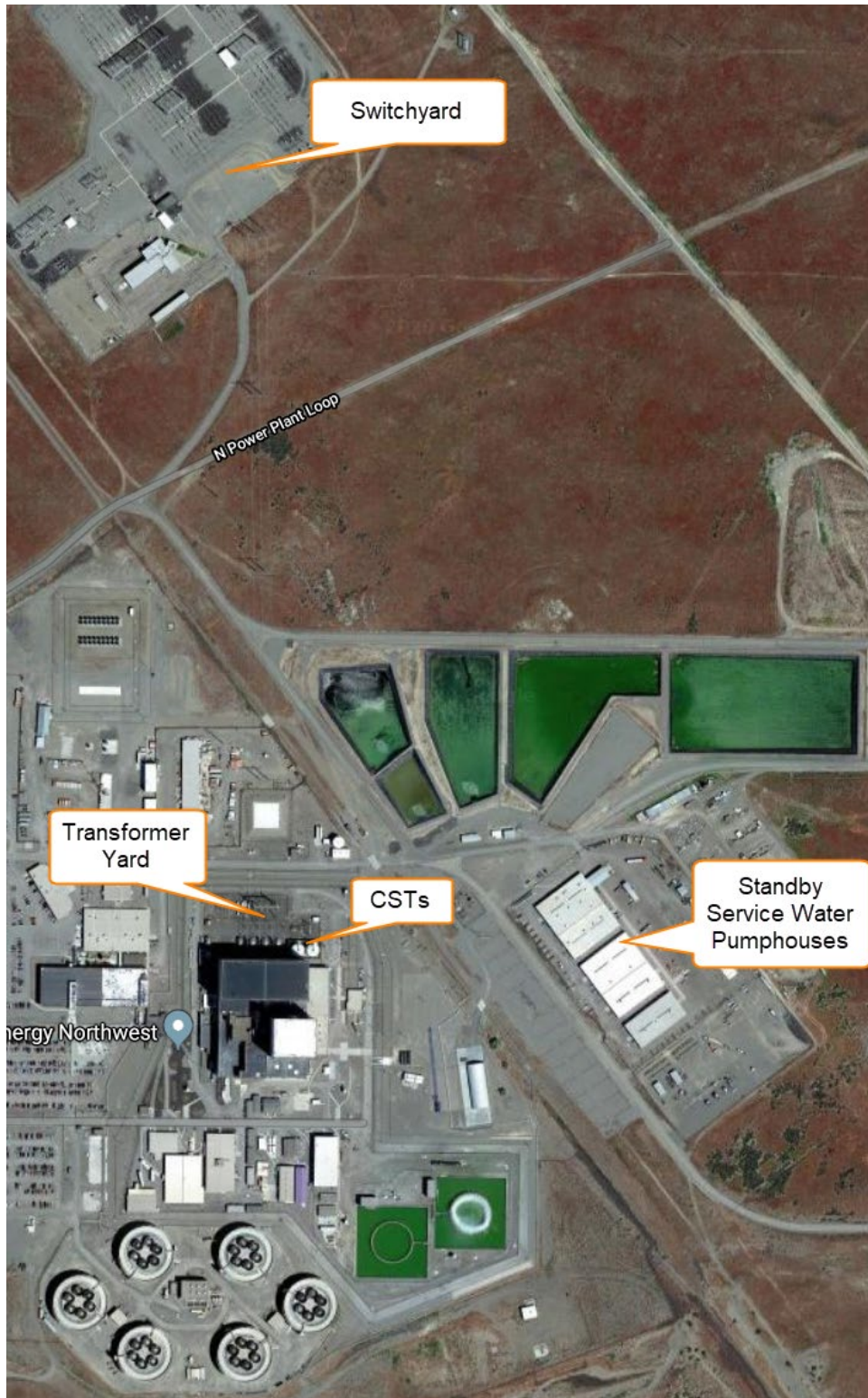
Figure 5-6. Columbia NPP site overhead view © Google Maps, Maxar Technologies, USDA.
