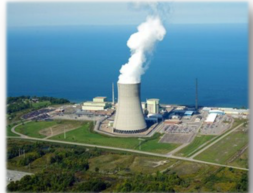
Nine Mile Point (Courtesy of Exelon)
