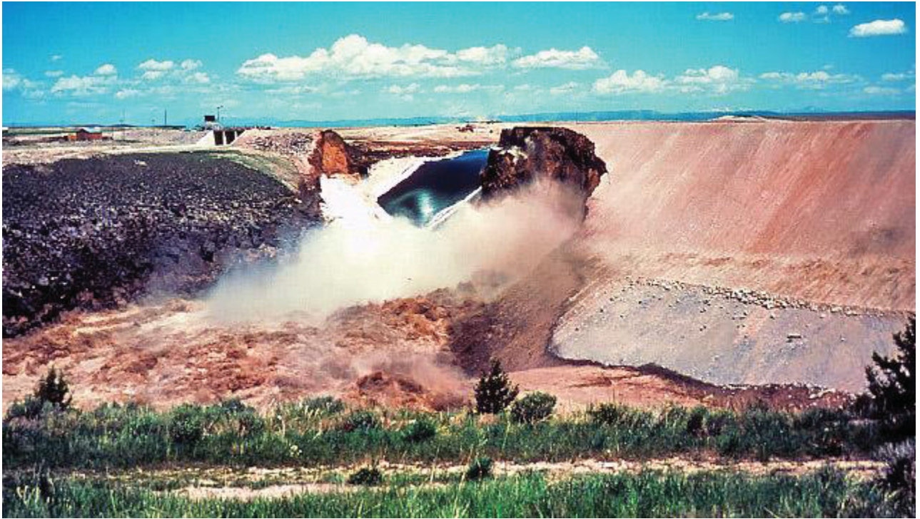
Figure 6. Teton Dam site showing complete failure
