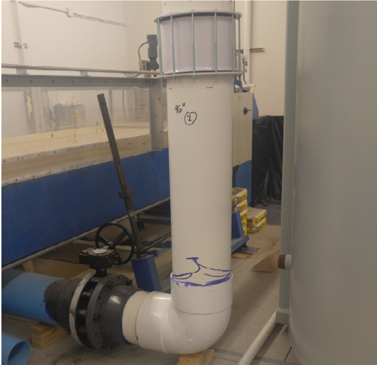
Figure 6. Existing 12-in pipe flanging with new piping installed.
