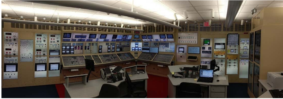
Figure 5. Robinson Nuclear Plant Glasstop Simulator Control Room.
