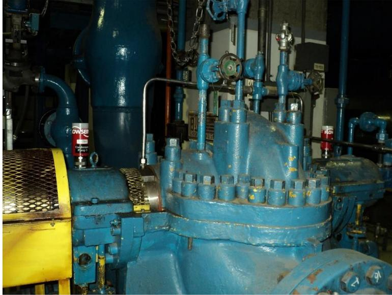
Figure 22. Installation of continuous monitoring integrated sensor-transmitter units on a condensate booster pump.
