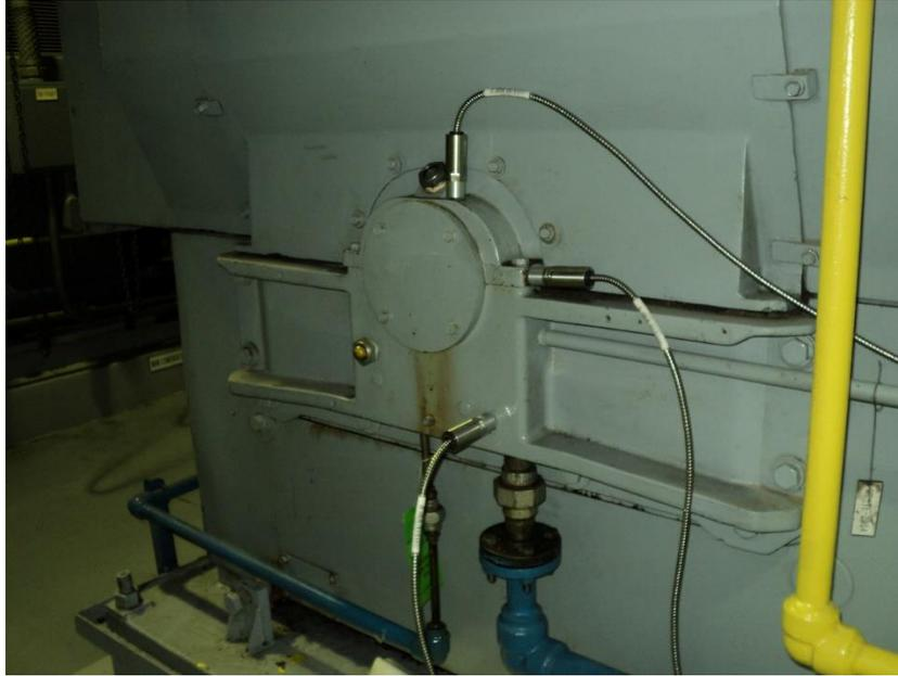
Figure 20. Installation of continuous monitoring vibration sensors on condensate booster pumps.
