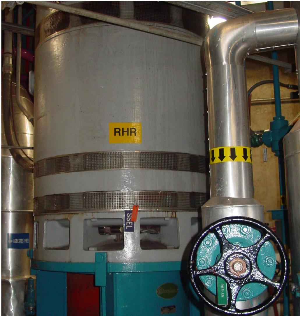
Figure 1. RHR pump picture at Cooper Nuclear Station.
