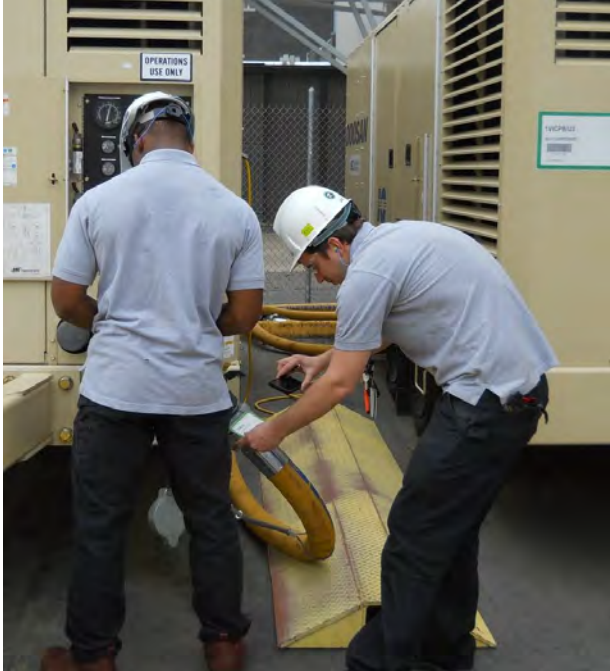
Figure 7. An AO Conducts a Digital CCV Using the CBP System.
