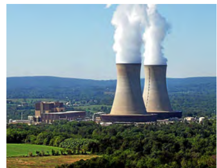
Limerick Generating Station
