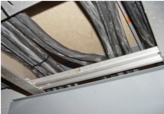
Figure 7.16. Twisted cable. Photo courtesy of EPRI.
