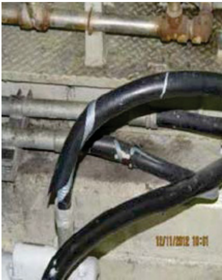
Figure 7.22. Ripped seal-tight on conduit near polyacrylic acid supply tank.
