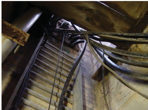
Figure 7.11. Poorly supported vertical runs. Photo courtesy of EPRI.
