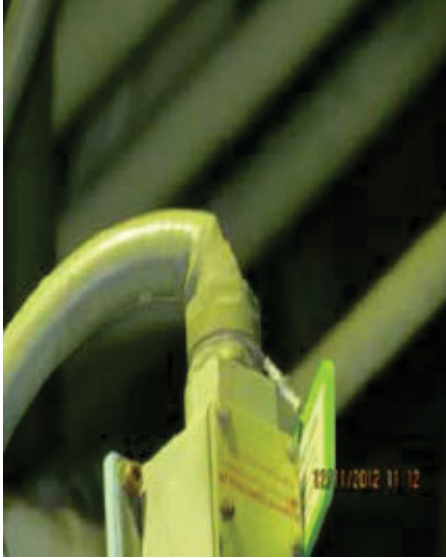
Figure 7.20. Very bent conduit entering a fitting near condensate polishing mixing bed service.
