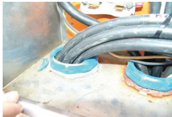
Figure 7.19. Contact with broken bushing. Photo courtesy of EPRI.
