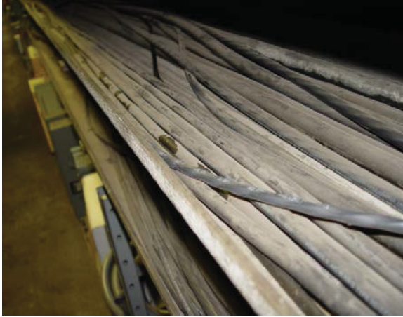
Figure 7.2. Full cable trays can make extraction of a single cable difficult and subject adjacent cables to damage. Photo courtesy of EPRI.
