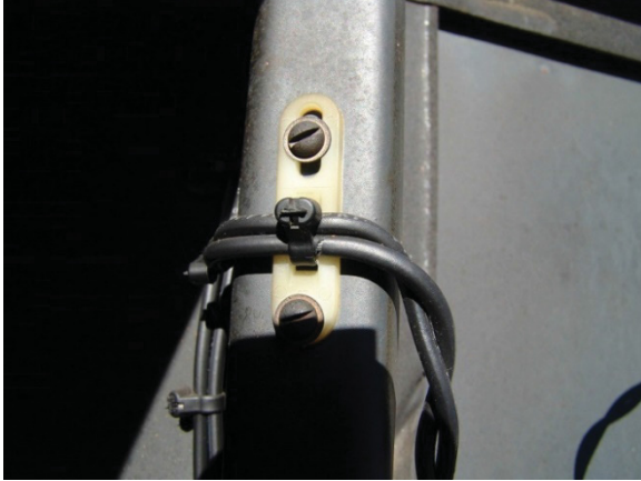
Figure 7.8. Excess cable tie tension. Photo courtesy of EPRI.
