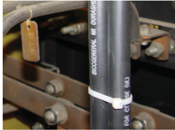
Figure 7.15. Cable ties constricting jacket and insulation. Photo courtesy of EPRI.
