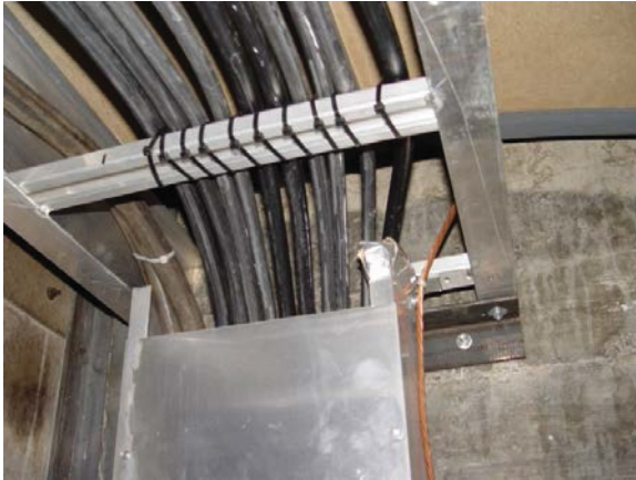
Figure 7.4. Cable contact along sharp edge. Photo courtesy of EPRI.
