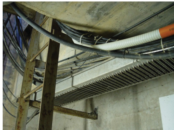
Figure 7.7. Unsupported cables outside of tray. Photo courtesy of EPRI.
