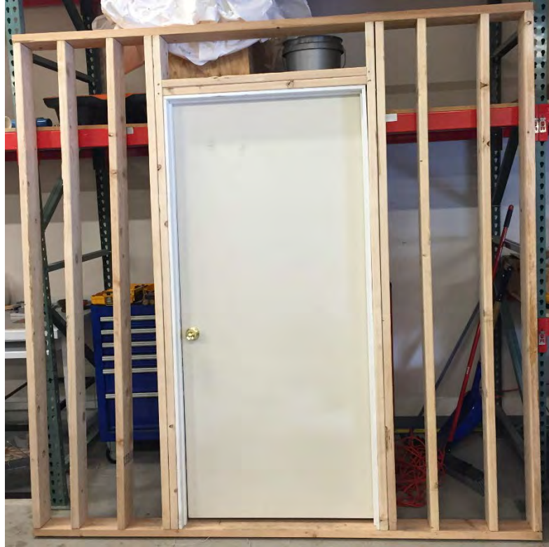
Figure 6. Wall frame and door assembly.
