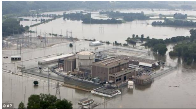
Figure 7. Actual Flooding Event.
