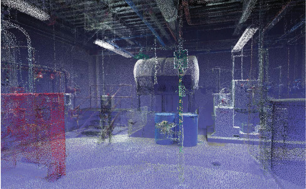
Figure 13: Point cloud of a chemical room taken using the Faro laser scanner.
