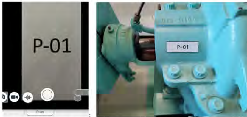
Figure 9. On the left: Depiction of the mobile phone's camera reading text (not an equipment label). On the right: Equipment tag at Xcel Energy for motor pump.
