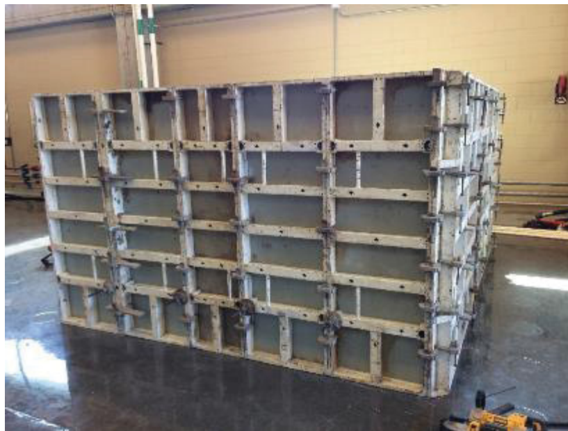
Figure 4.4- Fully constructed side formwork system
