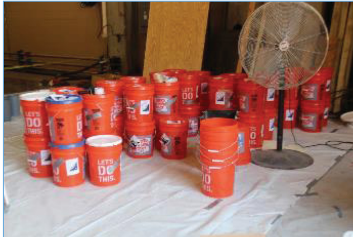
Figure 8.2- Diluted chemicals in buckets with tight-fitting covers
