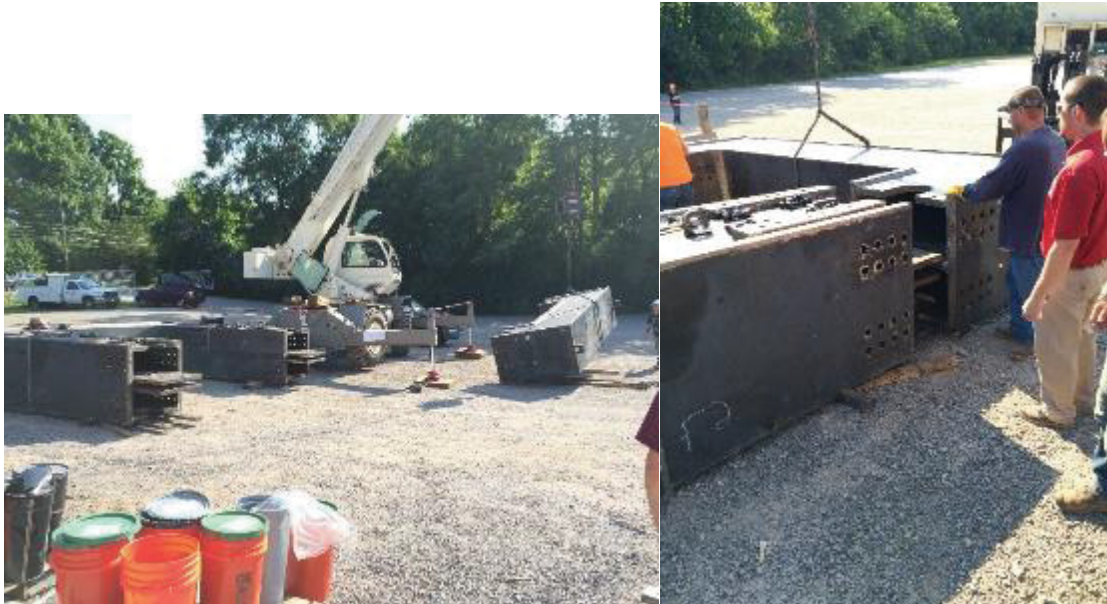
Figure 6.1- Demonstration of steel frame assembly
