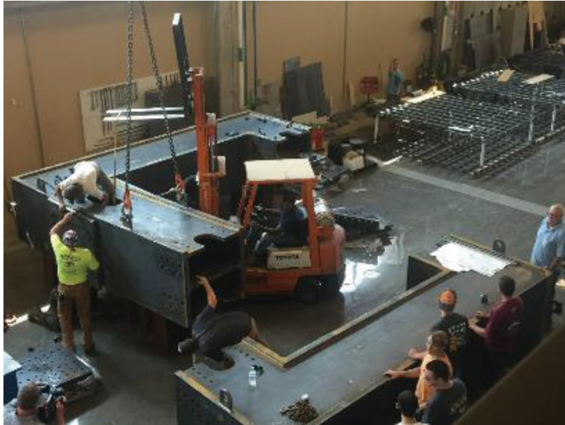
Figure 6.4- Steel Frame Assembly
