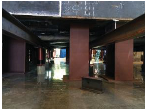
Figure 3.2- Painted steel supports in place
