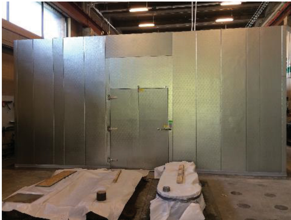
Figure 9.1- Completed side of chamber wall
