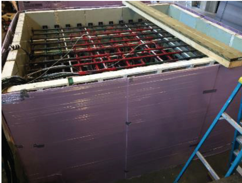
Figure 4.5- Completed installation of insulation around formwork
