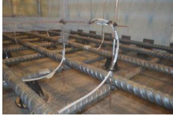
Figure 7.6- Installation of Fiber Optic Sensors in the passive length
