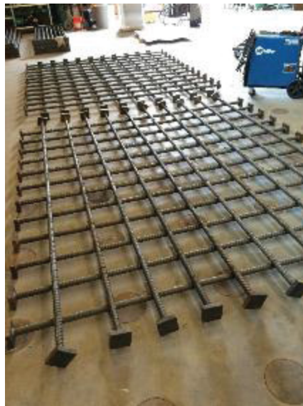
Figure 2.1- Completed construction of rebar layers
