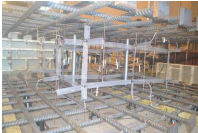
Figure 7.7- Installation of Fiber Optic Sensors
