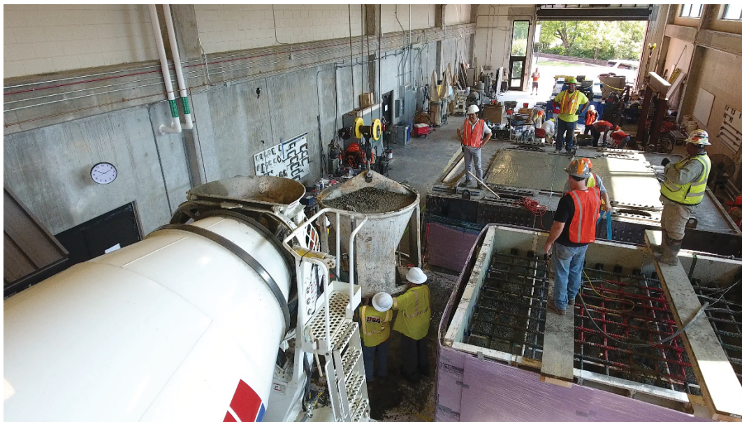
Figure 8.5- Filling concrete hopper from truck
