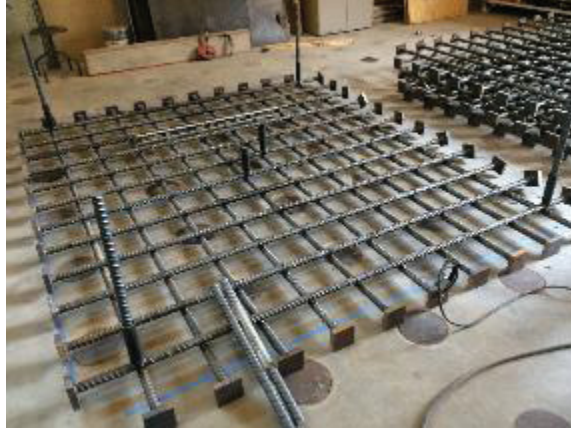
Figure 2.2- Installation of pipe sleeves and spacers
