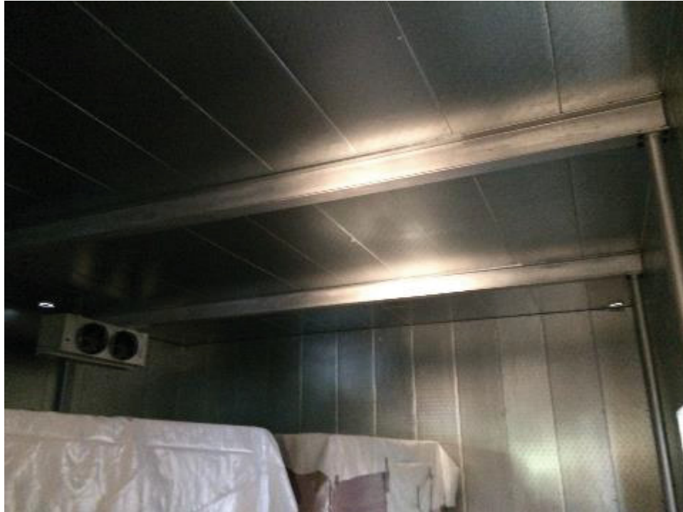
Figure 9.2- Completed ceiling before light installation
