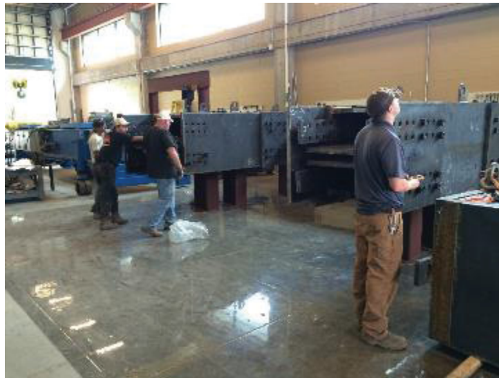
Figure 6.5- Steel Frame Assembly
