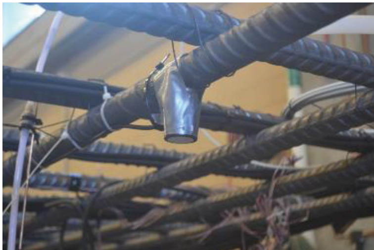
Figure 7.9- An acoustic emission sensor beneath the rebar
