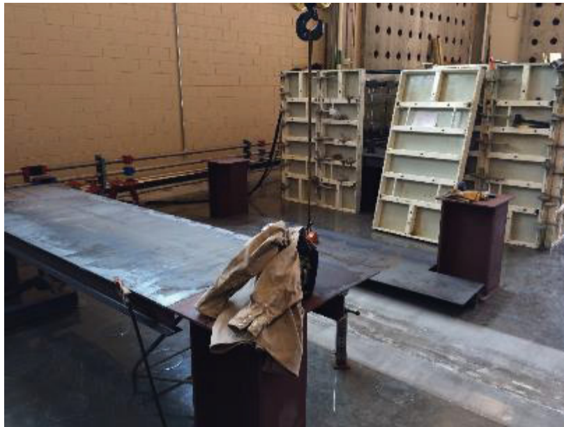
Figure 4.1- Edge pieces of bottom formwork being installed
