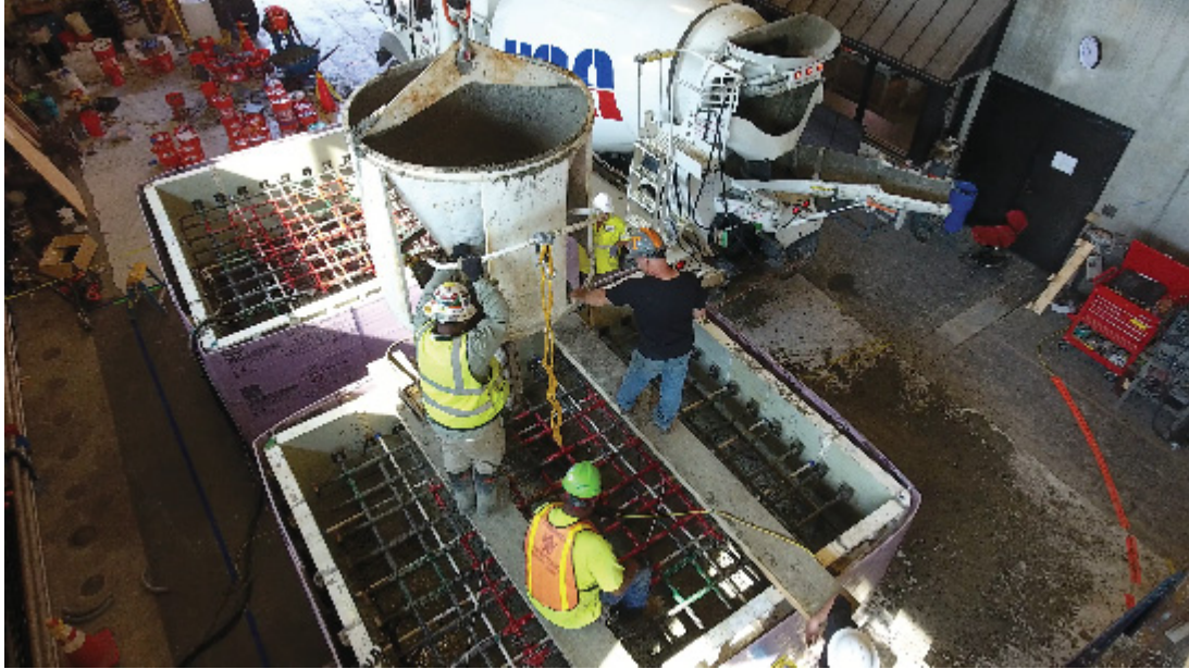
Figure 8.6- Placement of concrete
