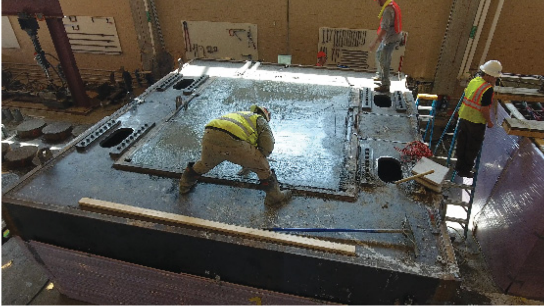
Figure 8.7- Finishing concrete surface
