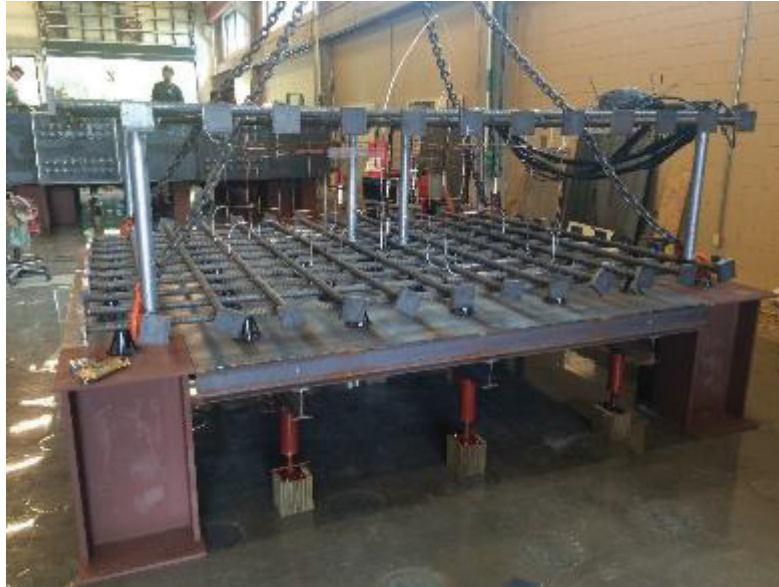
Figure 4.2- Completed construction of bottom formwork with cage in place
