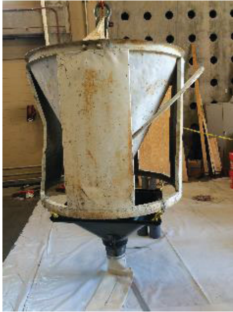
Figure 8.4- System of hoppers for concrete placement
