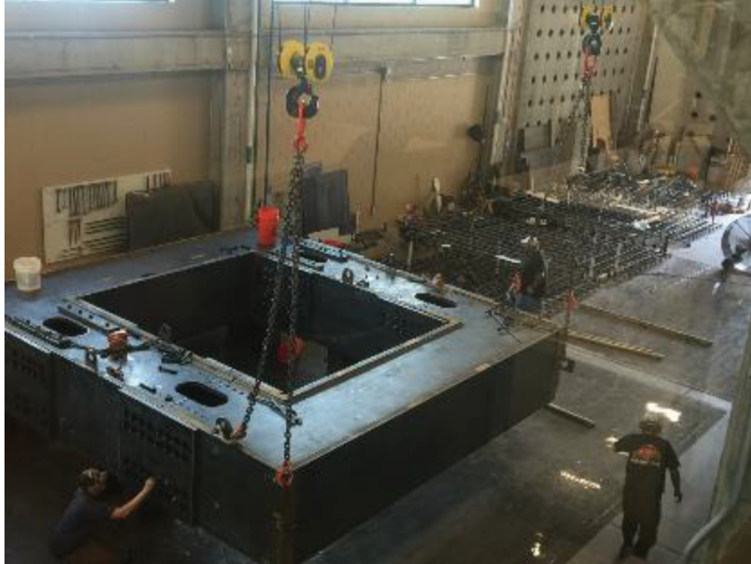
Figure 6.6- Steel Frame Assembly
