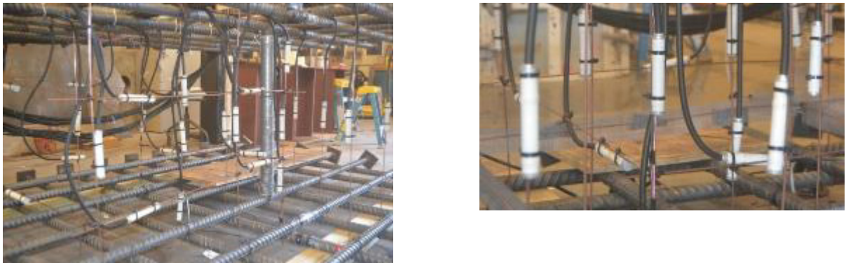
Figure 7.1- Installation of KM Sensors in the cages
