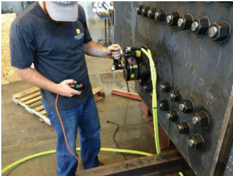
Figure 6.7- Steel Frame Assembly
