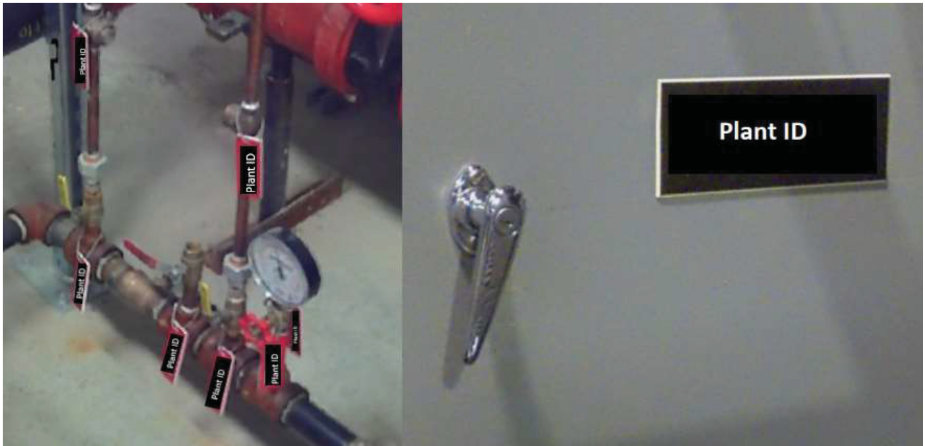
Figure 21. Equipment tags and placards used by nuclear facilities.
