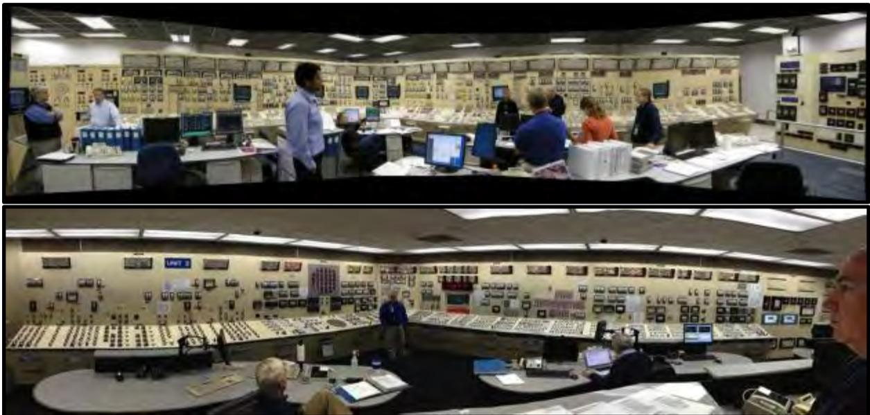
Figure 24. Actual Training Simulators Modeled on the Glasstop Panels.
