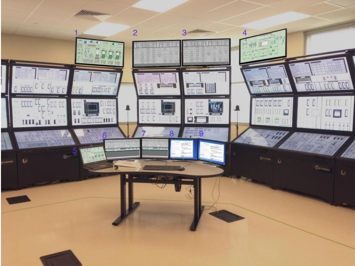
Figure 3. Mock-up Showing Potential Location of CPS Displays (8 & 9) on the SRO Workstation
