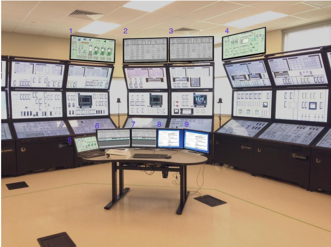
Figure 12. Mock-up Showing Proposed Location of HRP Task-Based Overview Displays (1, 4, & 5) in the HSSL
