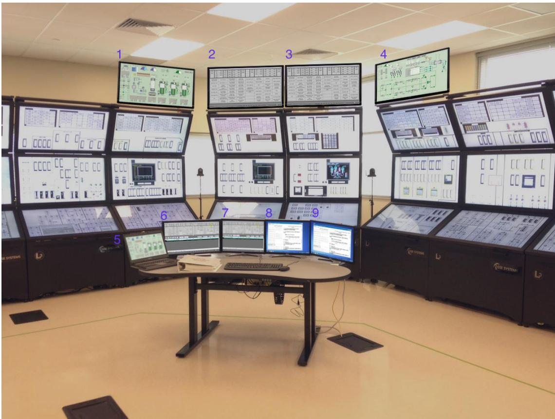
Figure 6. Mock-up Showing Proposed Location of APS Workstation Client (6 & 7) on the SRO Desk and APS Wall Panel Clients (2 & 3) in the HSSL.
