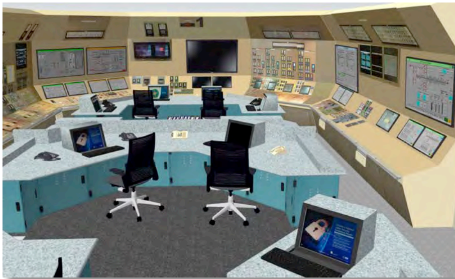
Figure 11. 3D model of the Palo Verde end-state concept for a hybrid control room.
