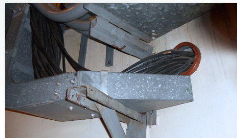
Figure 7. Low voltage cabling located near a reactor coolant pump inside Zion Station Unit 2 containment.
