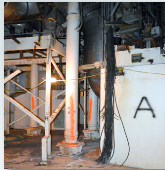
Figure 7. Low voltage cabling located near a reactor coolant pump inside Zion Station Unit 2 containment.
