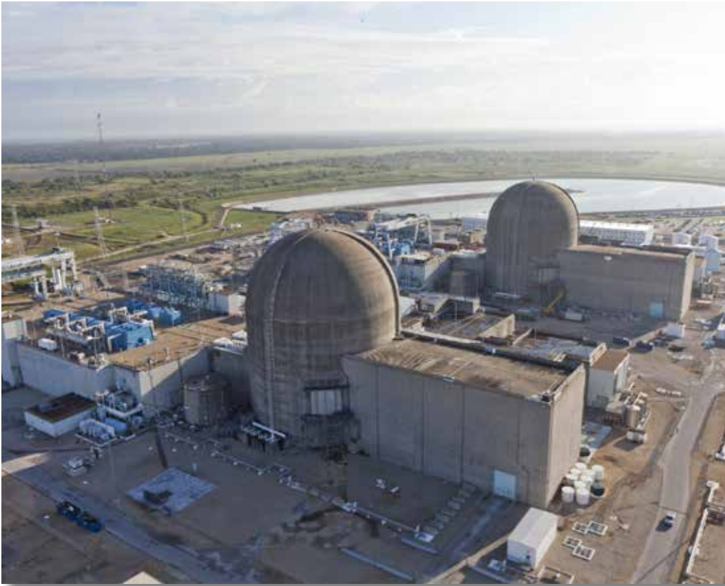
Figure 30. South Texas Project Nuclear Units.
