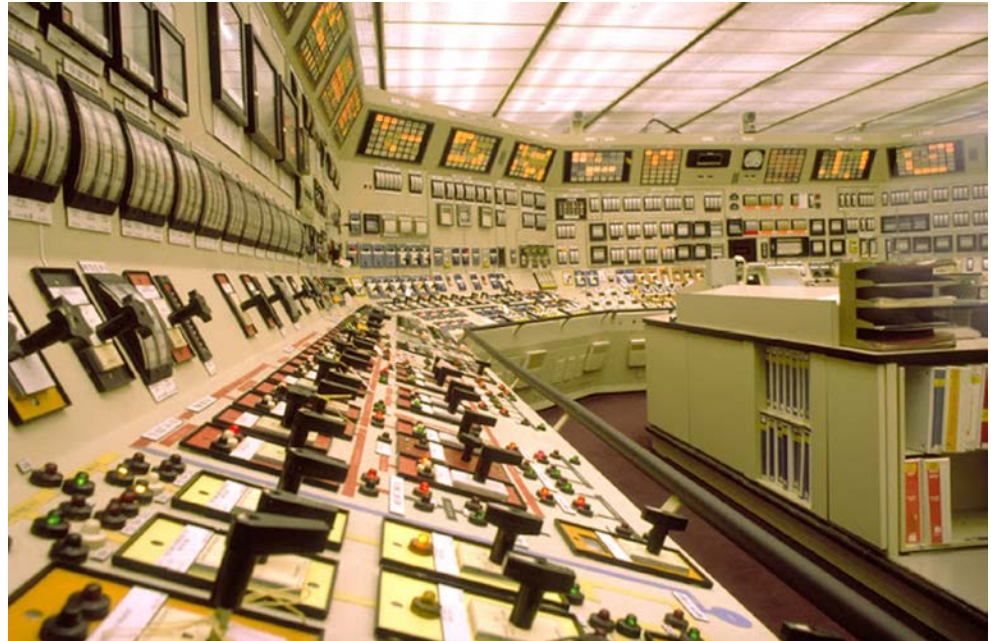
Figure 28. Much of the current instrumentation and controls in a nuclear power plant control room is analog technology.
