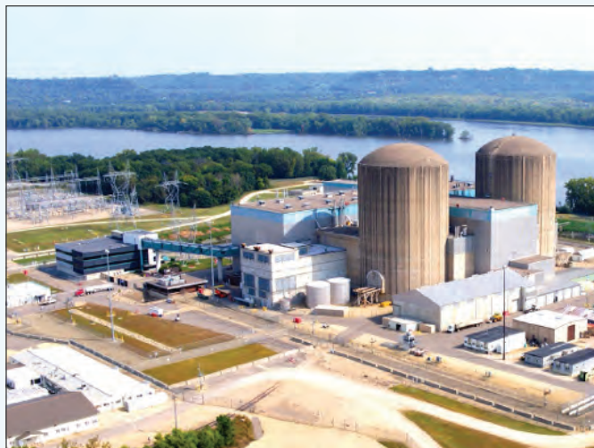
Figure 8. Prairie Island Nuclear Generating Plant in Welch, Minnesota
