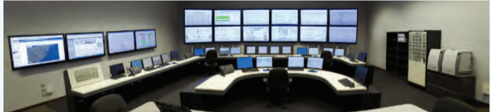
Figure 5. Photo of AP1000 nuclear power plant control room simulator used to train reactor operators.
