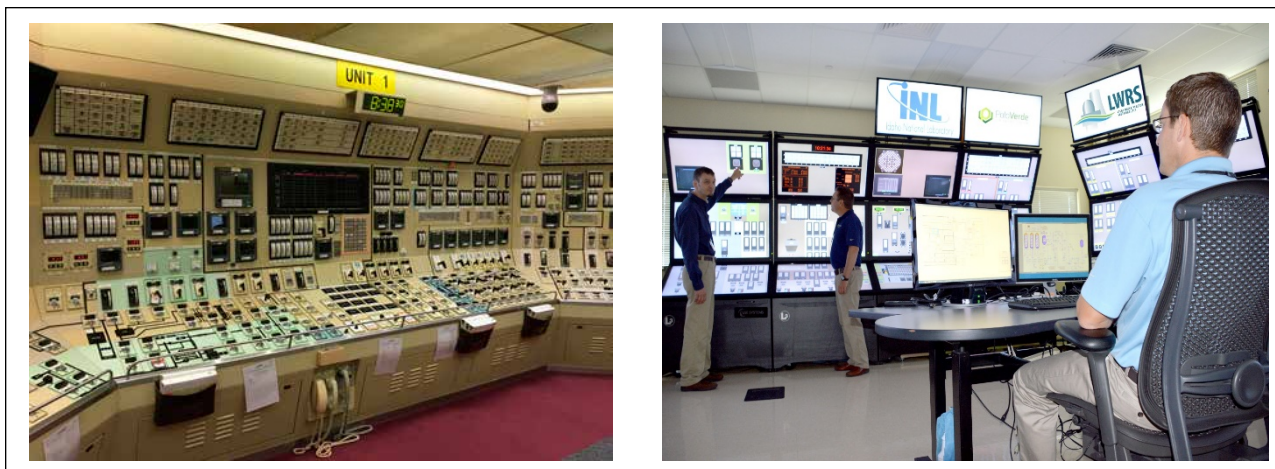
FIGURE 1 Left : Characteristic instrumentation in a nuclear power plant control room is dominated by analog technology. Right : Palo Verde operators participate in a control room modernization workshop in the Human Systems Simulation Laboratory at Idaho National Laboratory. Reprinted with permission from LWRS (2020).
