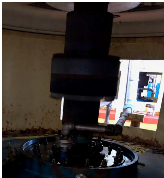
Figure 27. A rigid flanged coupling as taken from [21] (left) vs. a picture of the CWS shaft coupling (right).
