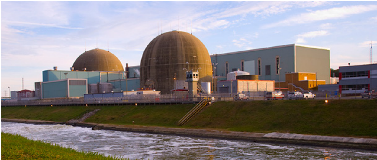
Figure 2-1. Photo of the Surry plant.[Reference 13].
