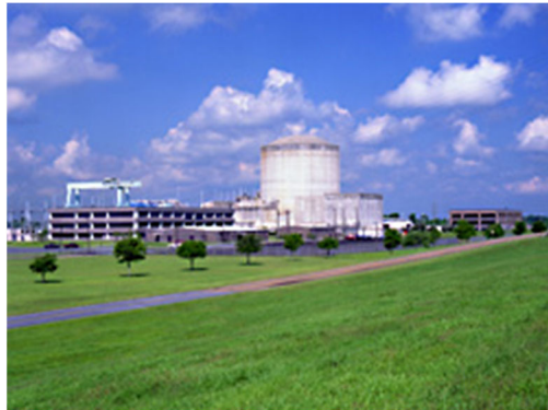
Figure 2. Waterford Steam Electric Station, Unit 3.
