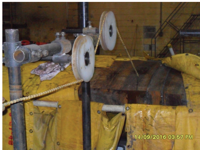
Figure 13. Wire saw cuts parallel to the beltline weld.
