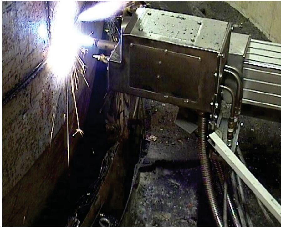
Figure 5. Vertical cut using an oxy-propane torch of a Zion Unit 1 RPV Level 2 Segment [11].
