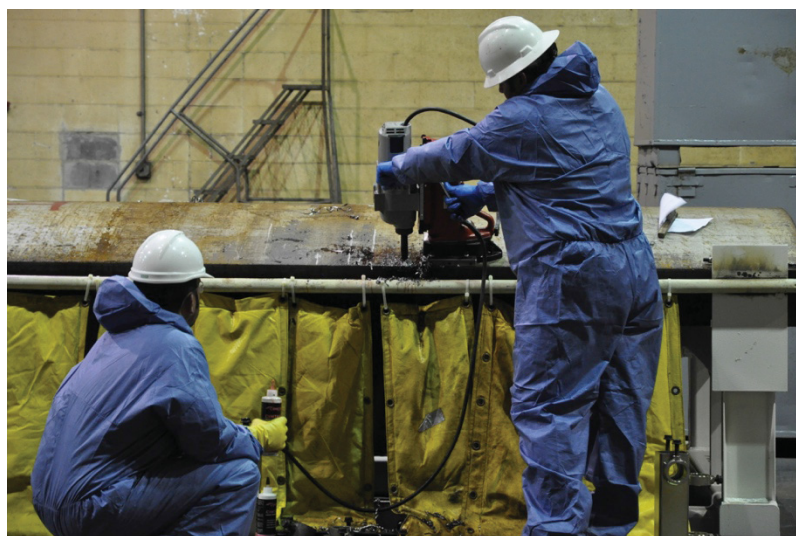
Figure 9. Drilling holes for wire saw to cut fresh surfaces to identify the beltline.
