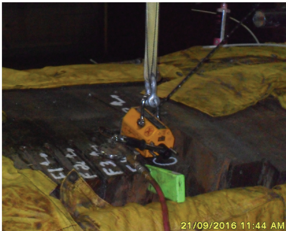
Figure 15. Lift magnet used to remove the cut blocks.
