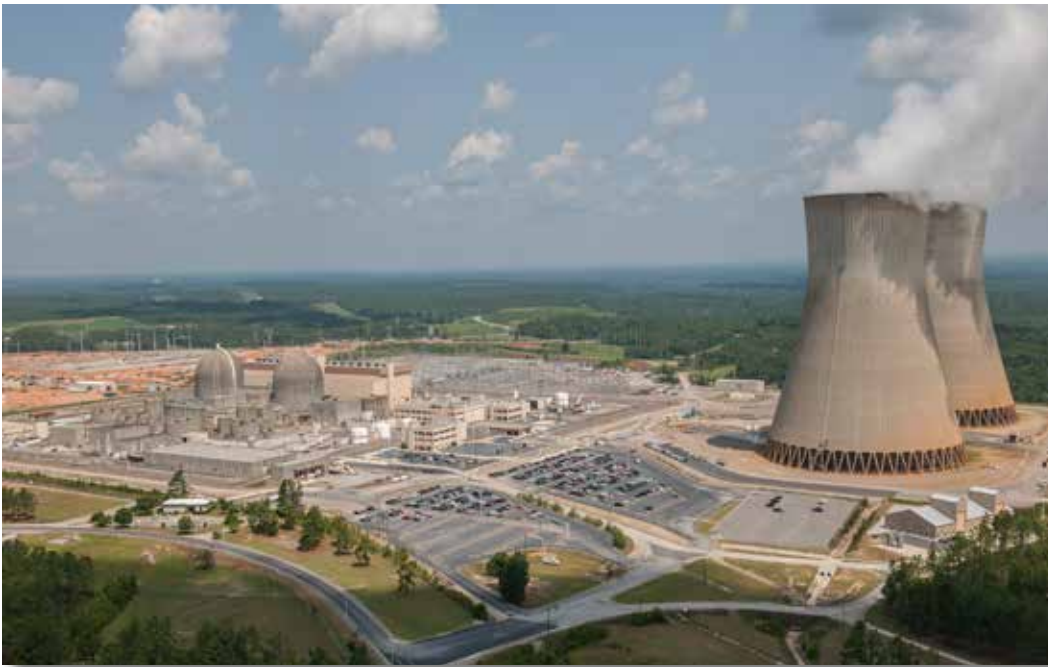
The Alvin W. Vogtle Electric Generating Plant, also known as Plant Vogtle, is a 2-unit nuclear power plant near Waynesboro, Georgia, is a partner in an LWRS Program pilot project on the Advanced Outage Control Center
