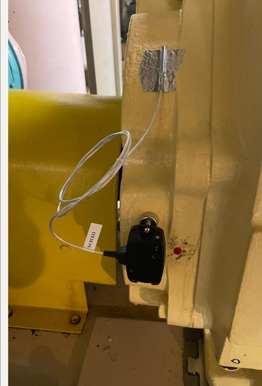
External Temperature and Vibration Sensor
