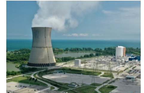
Vistra : Davis-Besse Plant
