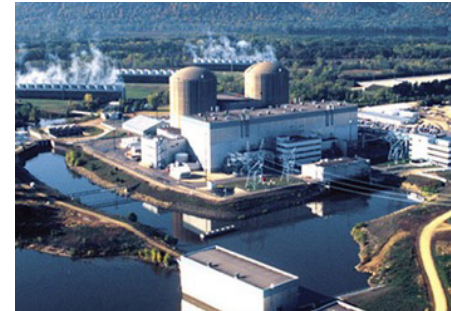
Xcel Energy: Prairie Island Plant
