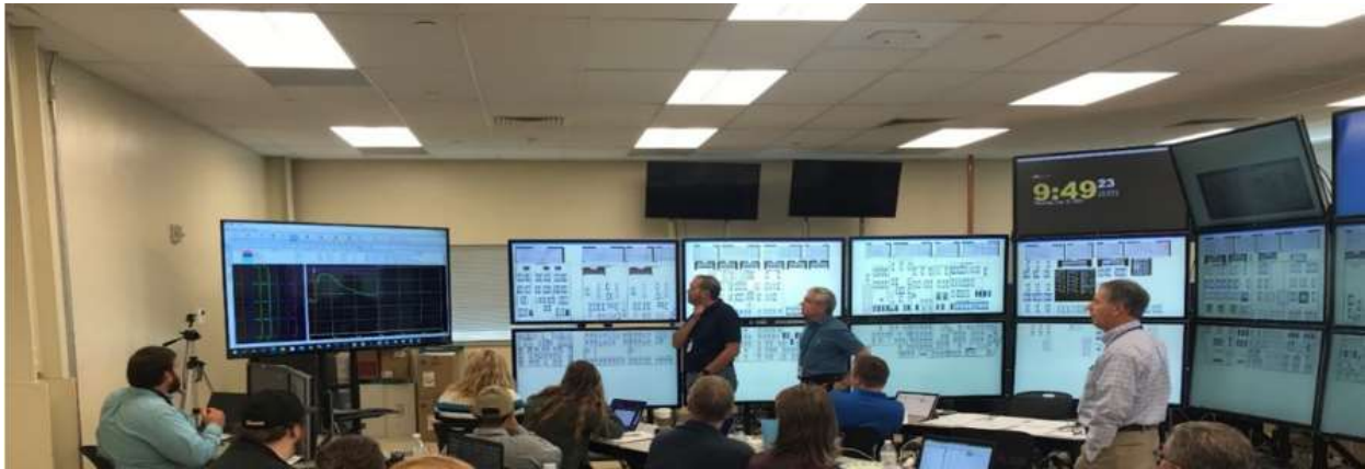
Figure 1. HSSL with virtual touch screens used to reproduce virtual analog control panels to support thermal power dispatch (TPD) scenarios.
