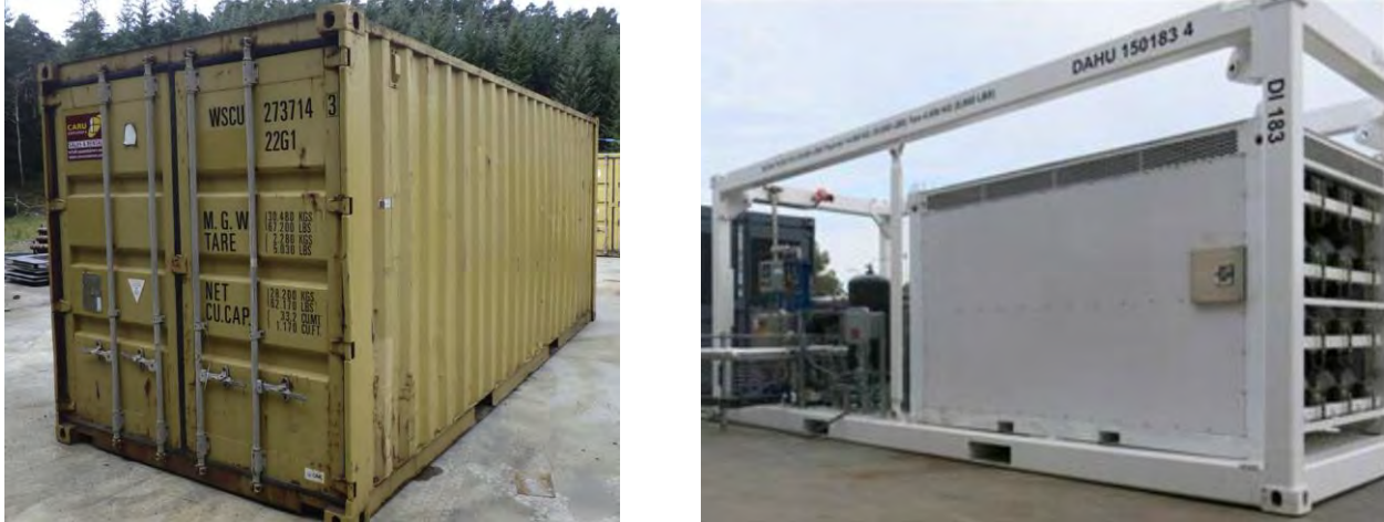
Figure 6-28. Shipping container as an SOEC's sealed enclosure (left) [24] and an open enclosure (right) [25].
