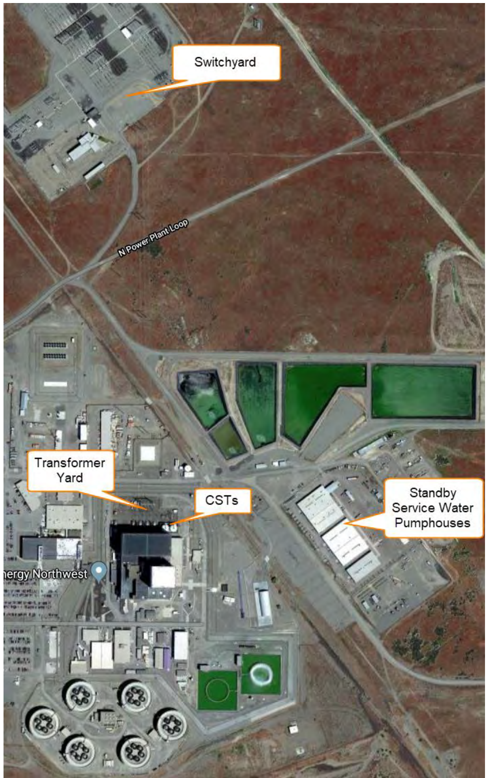
Figure 5-6. Columbia NPP site overhead view © Google Maps, Maxar Technologies, USA.
