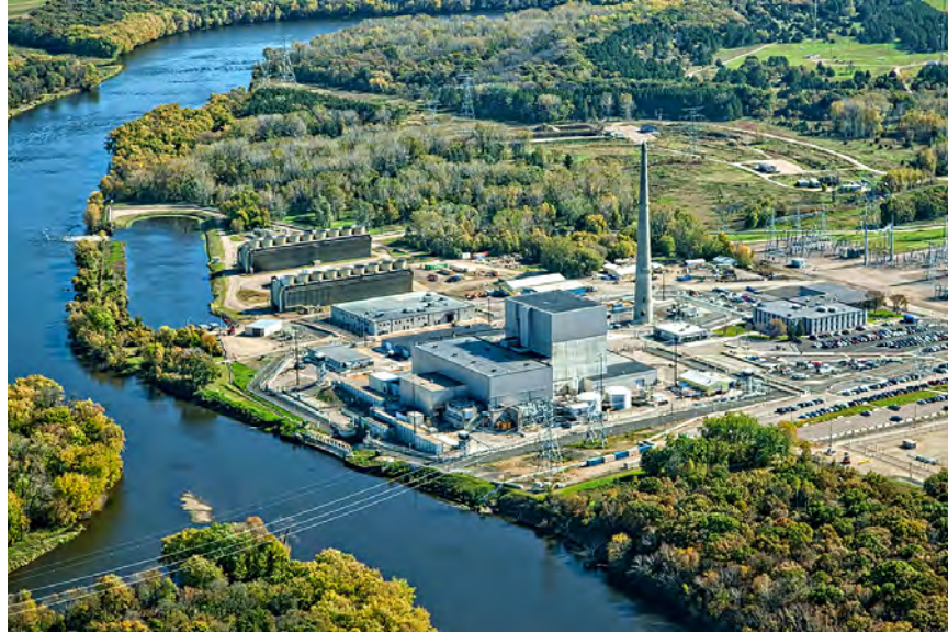
Figure 23. Monticello Nuclear Generating Plant in Monticello, Minnesota.
