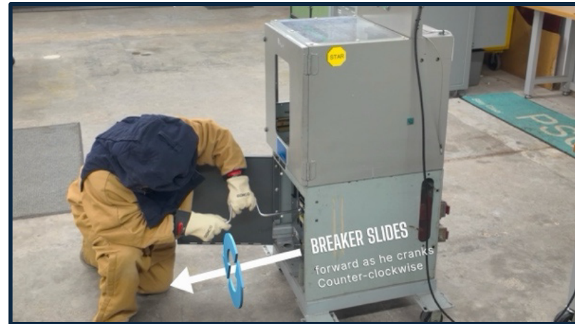
Figure 7. Use of special effects and graphics to enhance understanding. CBT video screenshot of testing (left), on-demand video screenshot of racking the breaker (right).
