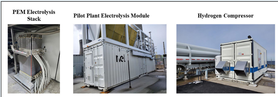
Figure 11. Nel PEM water electrolysis stack, pilot plant electrolysis module and hydrogen compressor.
