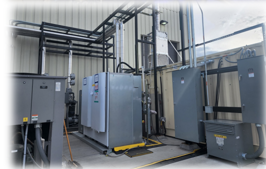
High Temperature Electrolysis (Bloom 150 kW Module)
