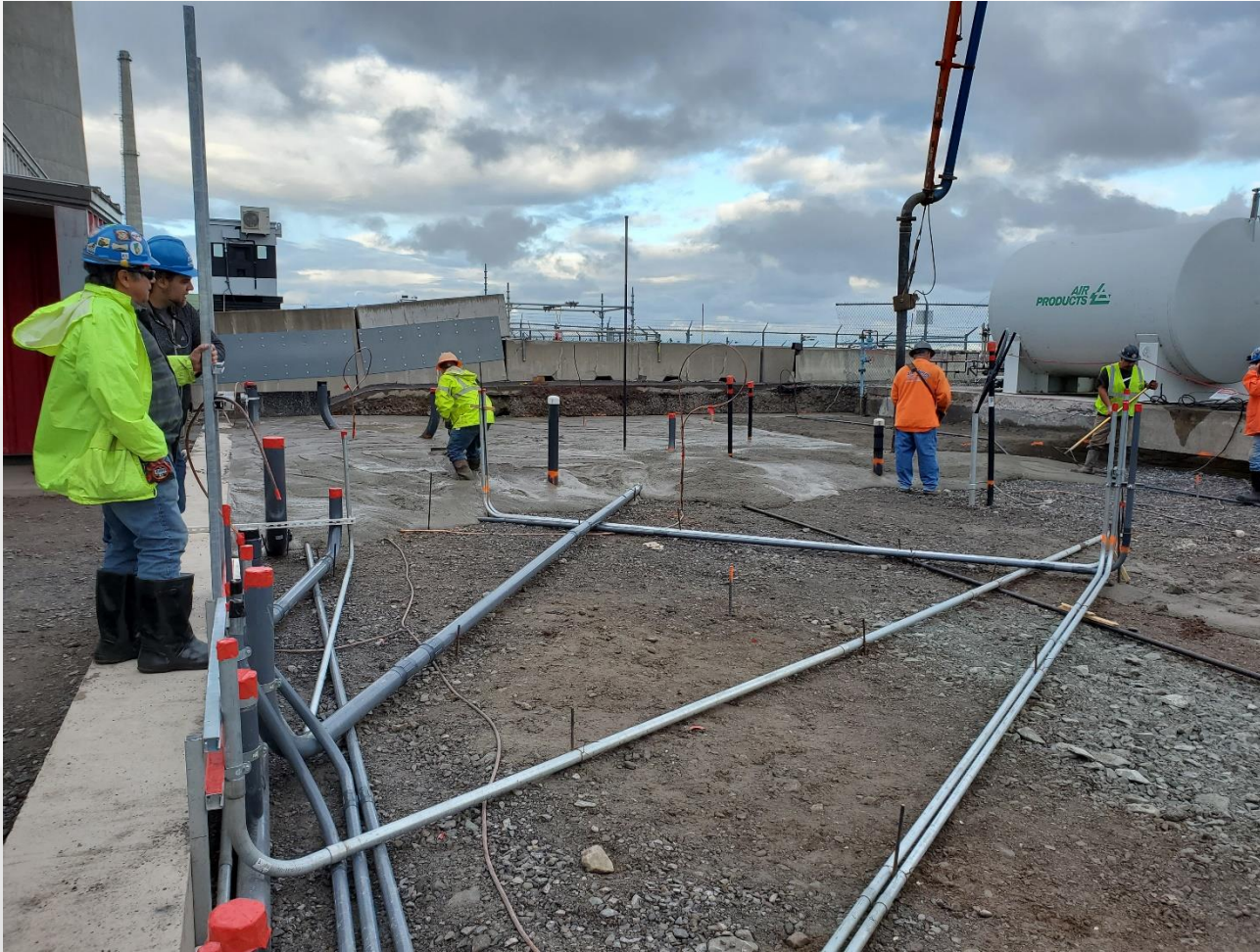
Pouring concrete for electrolyzer on left, rigging power supply into place on right
